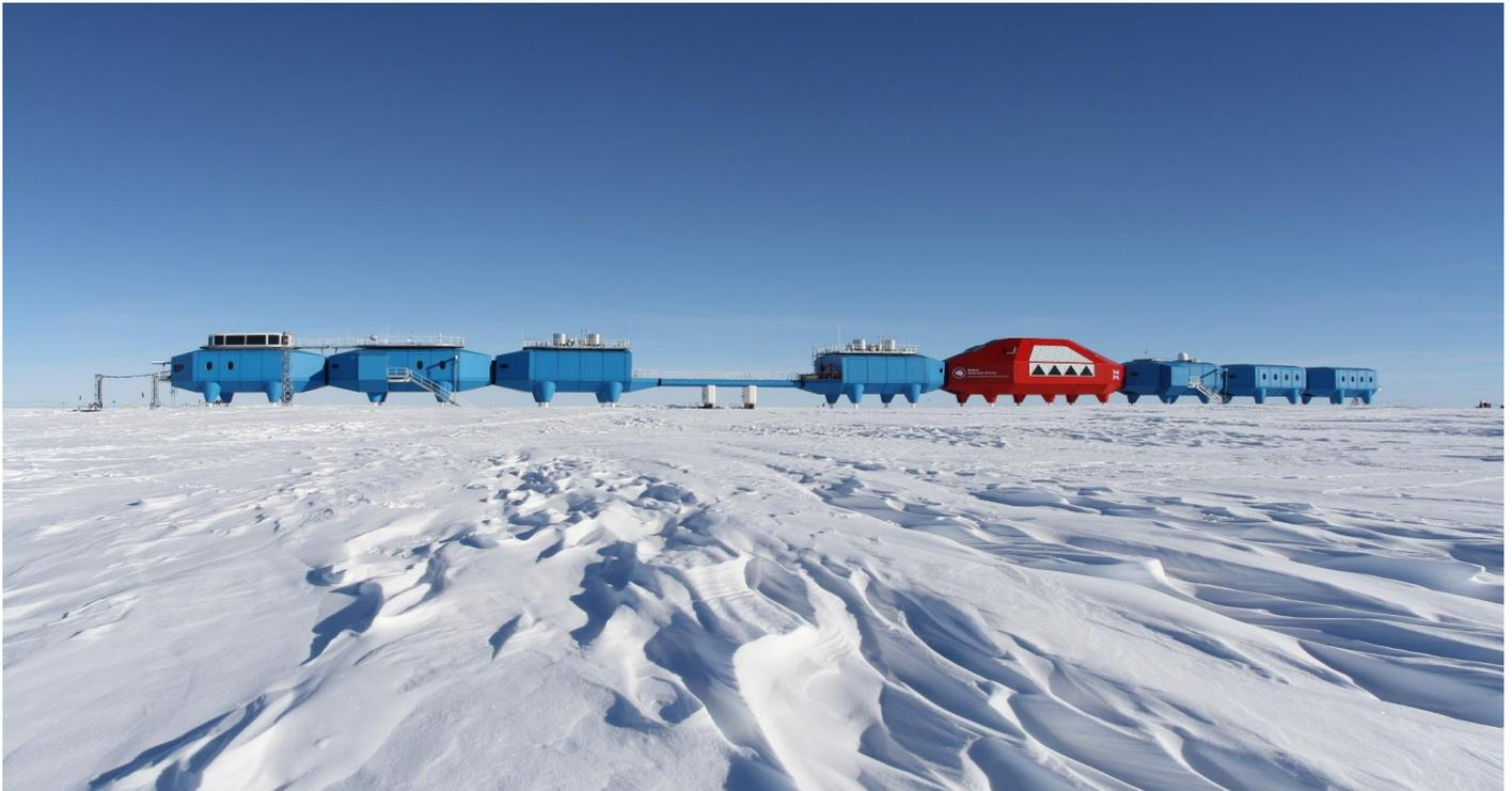
Halley VI, the British Antarctic Survey's new 'space-age' Antarctic research station, is one of the most technically challenging projects ever delivered. Halley VI is designed to lift itself out of the snow to prevent it from being buried by the ever-increasing snow accumulation and has the ability to be relocated to avoid an unstable ice shelf that could potentially break up during its lifetime.
